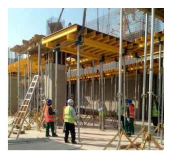
Varitable system for edge zones of a slab can be assembled in a way, that casting of drop-beams or stop-ends can be provided much easier, with all features integrated in one system.
